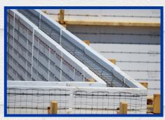
Quickly and easily secure Perma Form with its own bracing system that hooks directly into its wires.
